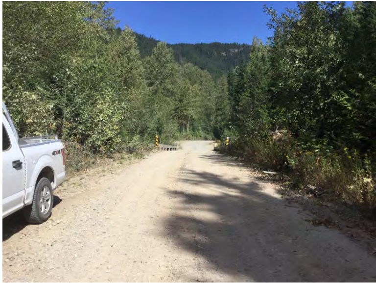
Approach from Right Bank when facing downstream
