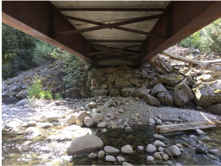
Right Bank Abutment when facing downstream
