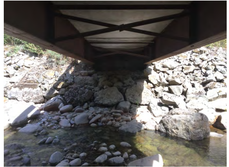
Left Bank Abutment when facing downstream
